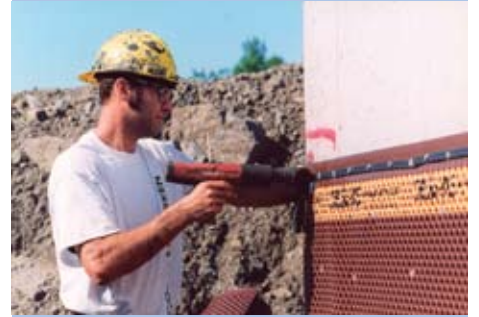
DELTA® - MS/DELTA® - TERMINATION BAR install
