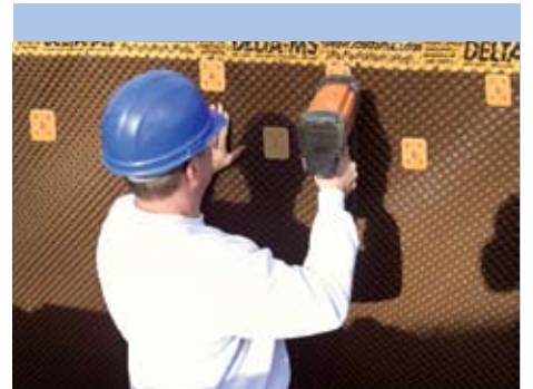
DELTA®- MS/DELTA®- FAST'ner install
