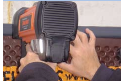
DELTA®- MS/DELTA®- FLASH install
