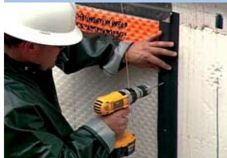
DELTA® - MS CLEAR/DELTA® - MOLD STRIP install
