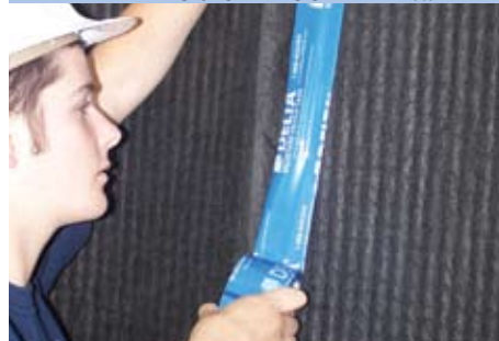
DELTA®- DRAIN 6000/ DELTA®MOISTURE PROOF TAPE install
