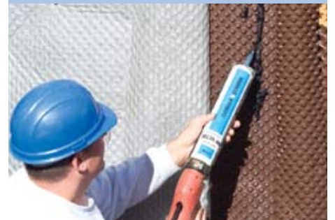
DELTA®- DRAIN/DELTA®- SEALANT install
